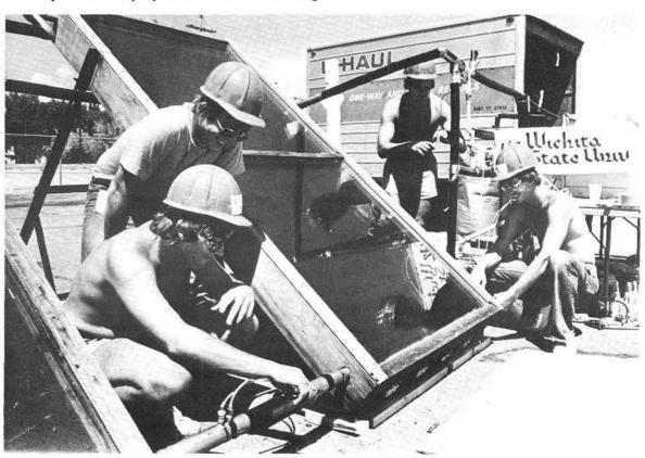
WICHITA STATE solar collectors are designed to provide space heating.
